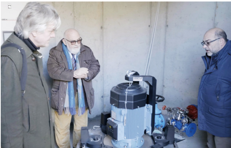
Mayor Avernino di Croce and engineer Antonino Basile explain the Pelton 20 kW turbine in Venaus.
